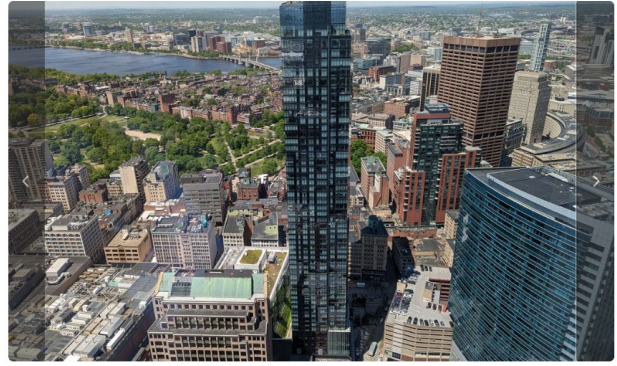
The Millennium Tower, built by the same developer as Winthrop Center in 2016, stands a few blocks west up Franklin Street.
