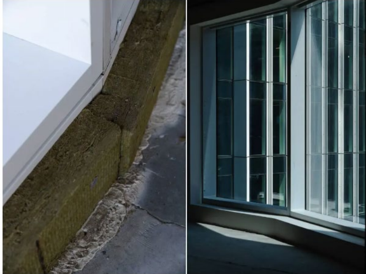
Insulation, left, lines the windows of the Winthrop Center. Sophie Park for The New York Times
